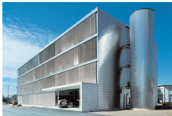
The new Franke holding company building
